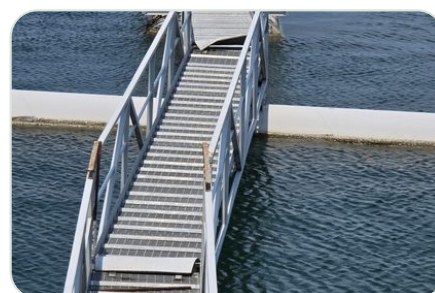
Walkway & gangway installation
