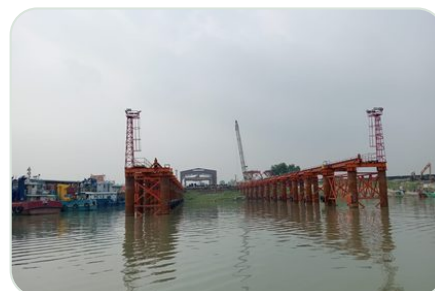
Jetty & steel structure works
